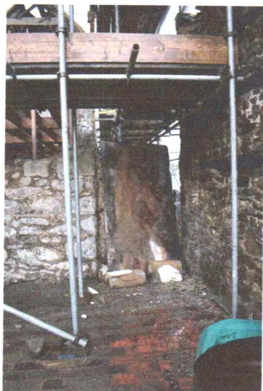
Fig. 5 and 6 Junction in wall where rear building adjoins front wing, showing as a dog leg on historic maps
