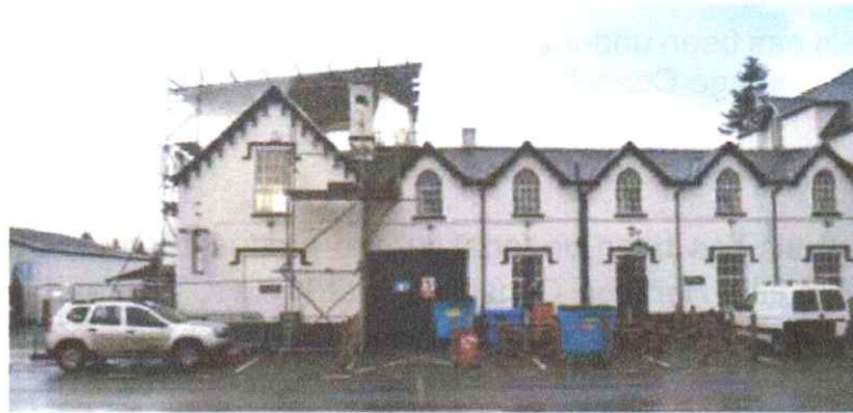
Former Coach House Former Assembly Rooms
